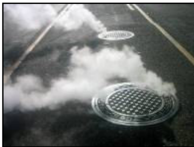
Leaking Traps Waste Energy
