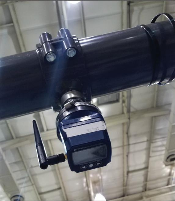
Figure 15 – Two WGRs installed on temperature gauges
