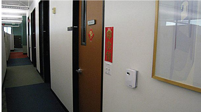
Figure 5: A WPT works with original equipment and controls like native DDC.
