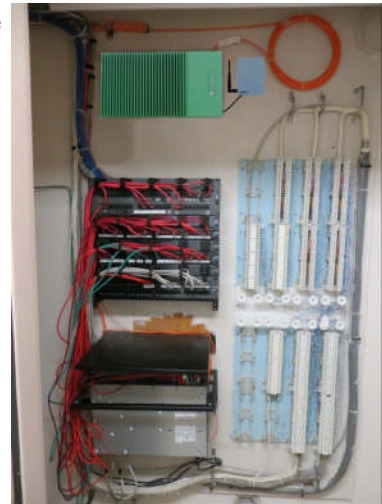
Control panel wiring linking the new thermostats back to the existing Building Automation System
