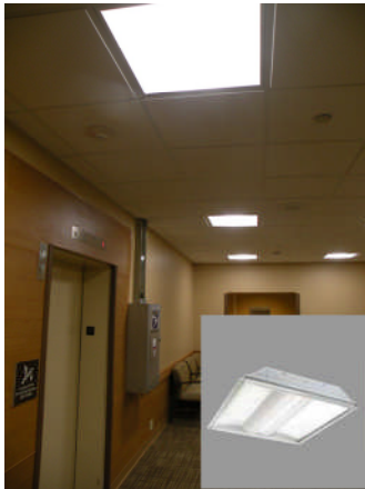
LED 2x2 Lensed Troffers in Elevator Lobby
