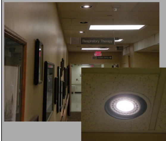
LED Par Lights used to highlight the Art Wall in Respiratory Therapy
