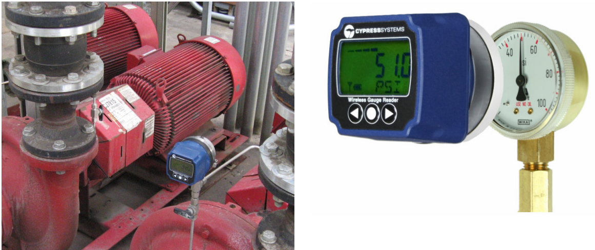
Figure 2 – Non-Invasive Mounting for Wireless Gauge Reader
