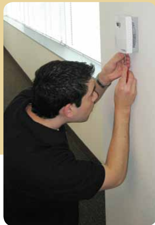
GOLD WINNER: Cypress Envirosystems' Wireless Pneumatic Thermostat (WPT) retrofits to existing pneumatic thermostats without rewiring to enable zone control.
