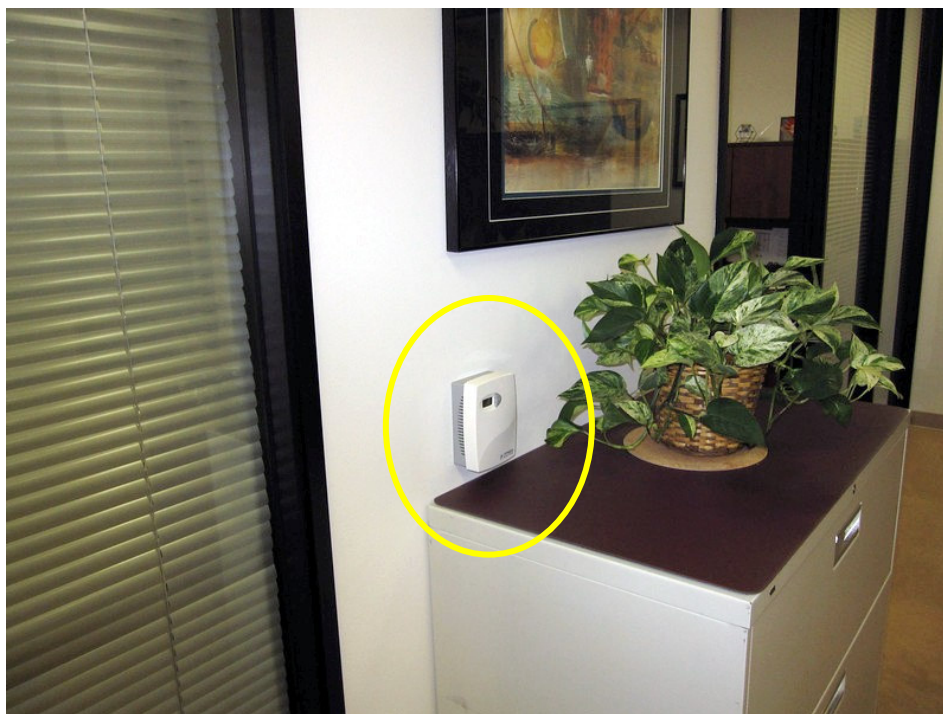
Figure III – Wireless Pneumatic Thermostat
