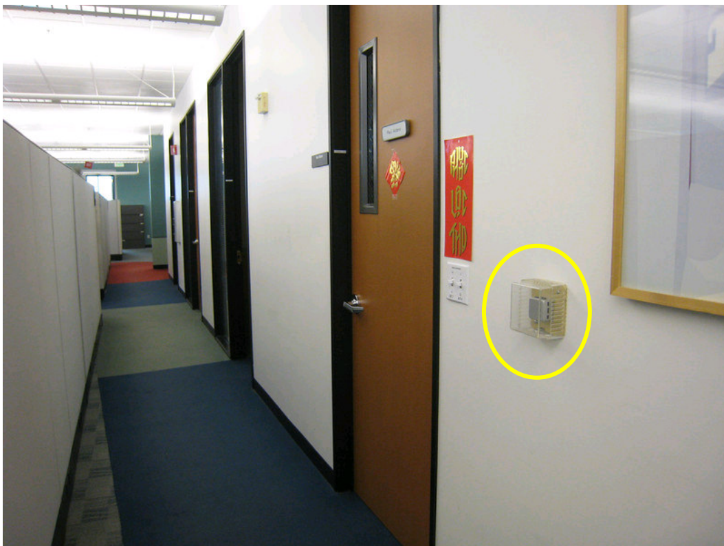
Figure II – Existing Pneumatic Thermostat prior to retrofit
