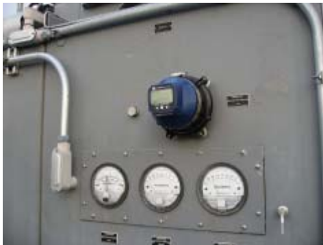
Wireless Magnehelic Reader Monitors Filters and Airflow
