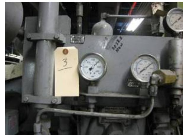
Hydrogen Dryer Tower Pressure
