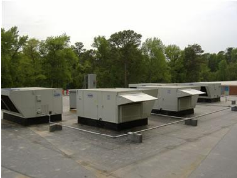
Typical Air Handler Units
