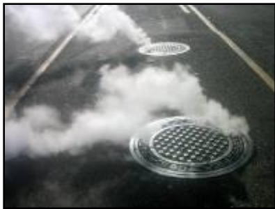
Leaking Traps Waste Energy
