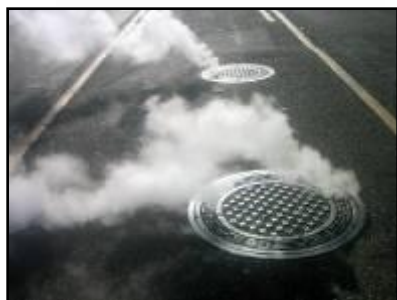
Leaking Traps Waste Energy
