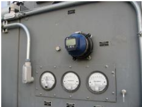
Wireless Magnehelic Reader Monitors Filters and Airflow
