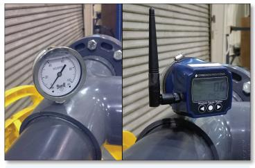
Figure 14 – WGR installed on pressure gauge
