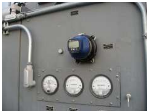
Wireless Magnehelic Reader Monitors Filters and Airflow
