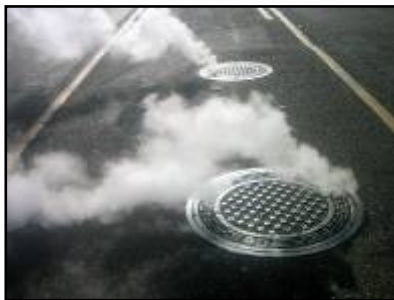
Leaking Traps Waste Energy
