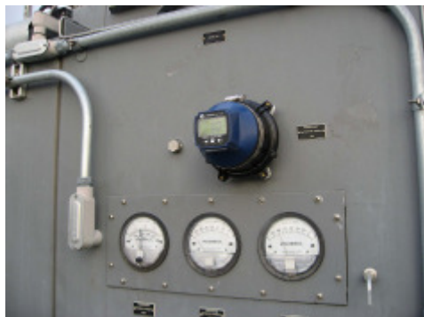
Wireless Magnehelic Reader Monitors Filters and Airflow
