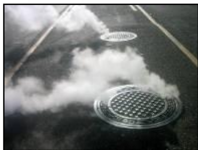
Leaking Traps Waste Energy
