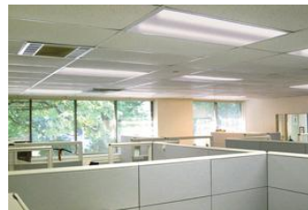
Legacy Fluorescent Lighting
