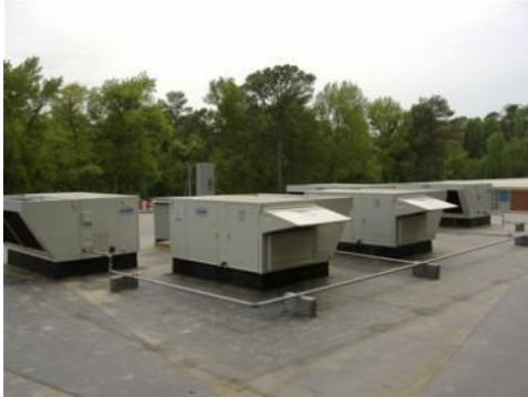
Typical Air Handler Units
