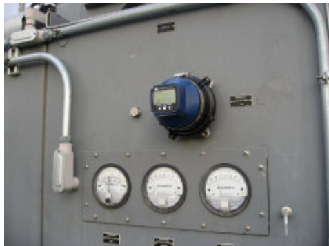
Wireless Magnehelic Reader Monitors Filters and Airflow
