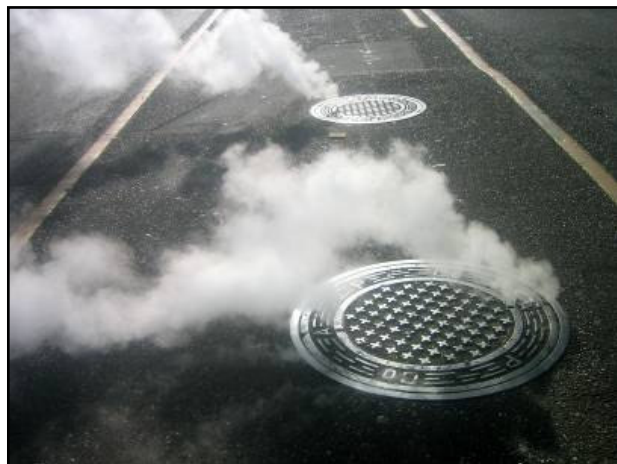
Figure 1 – Signs of a leaking steam trap
