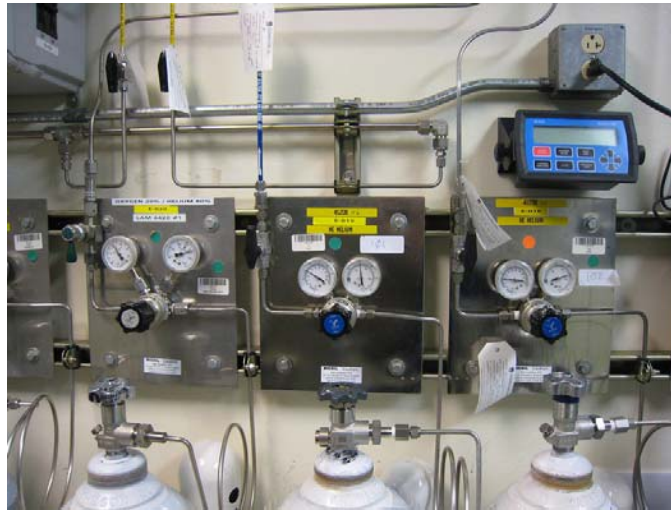
Figure 1 – Micrel Gas Cylinder Area (typical)
