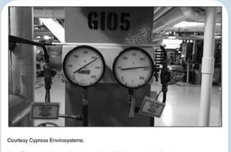
Note: Thousands of manual gauges monitor critical parameters such as pressure, temperature, and flow; the readings are not digitized and do not lend themselves to IoT o fault detection analytics.
