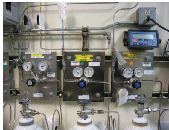
Figure 1. A typical Micrel gas cylinder area
