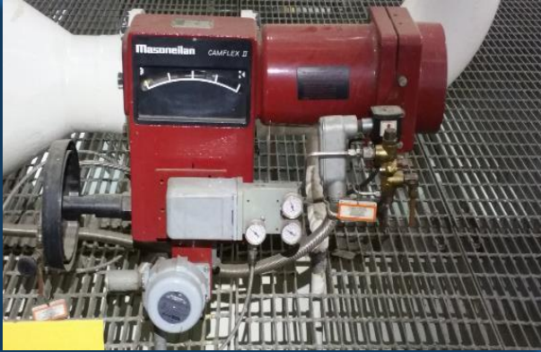
Air Operated Valve (AOV)
