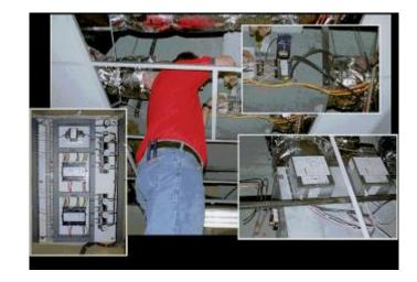
Upgrading from pneumatics to DDC is extremely labor intensive, costly, and disruptive to occupants
